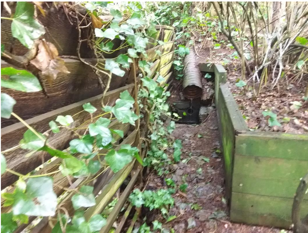
Figure 19. Looking east at the drainage system
