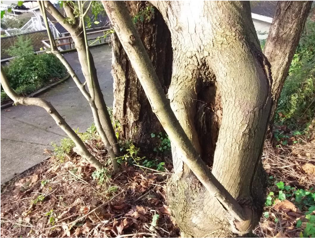
Figure 35. Decayed area at base of another of the #13 maple stems
