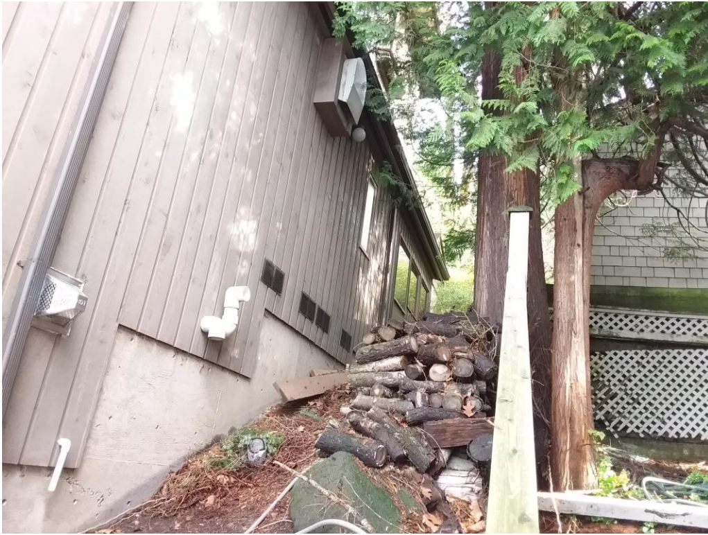
Figure 28. Looking east at the lower formation of the #8 cedar.
