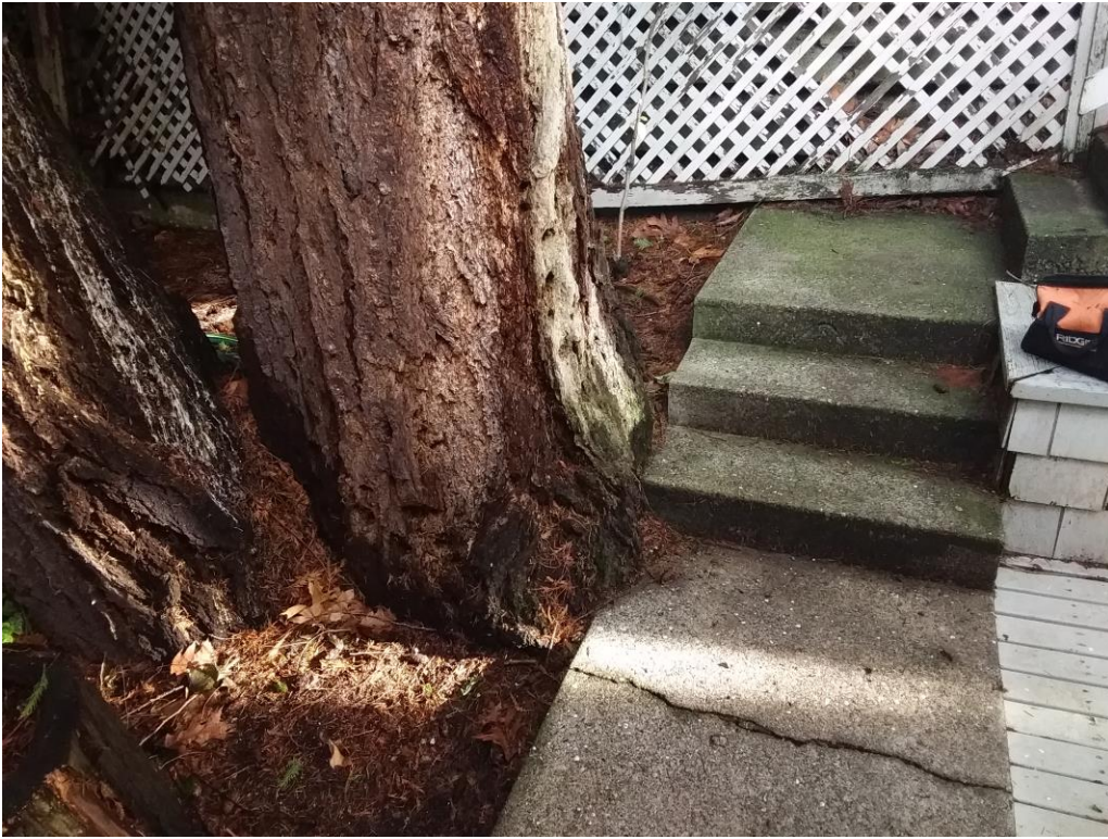
Figure 22. Looking down and east at the base of the #6 fir.
